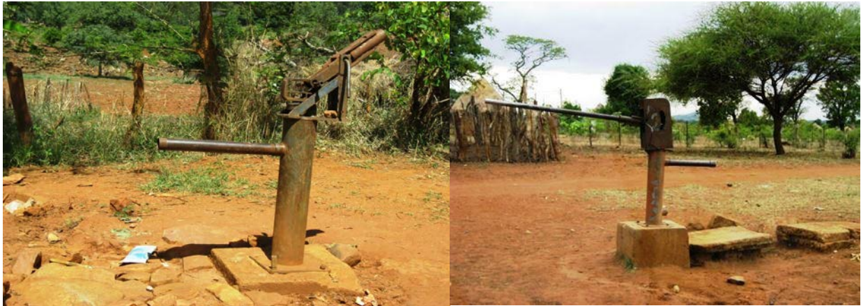
Figure 5: Non-functional hand-pumps or boreholes in Lambani.
